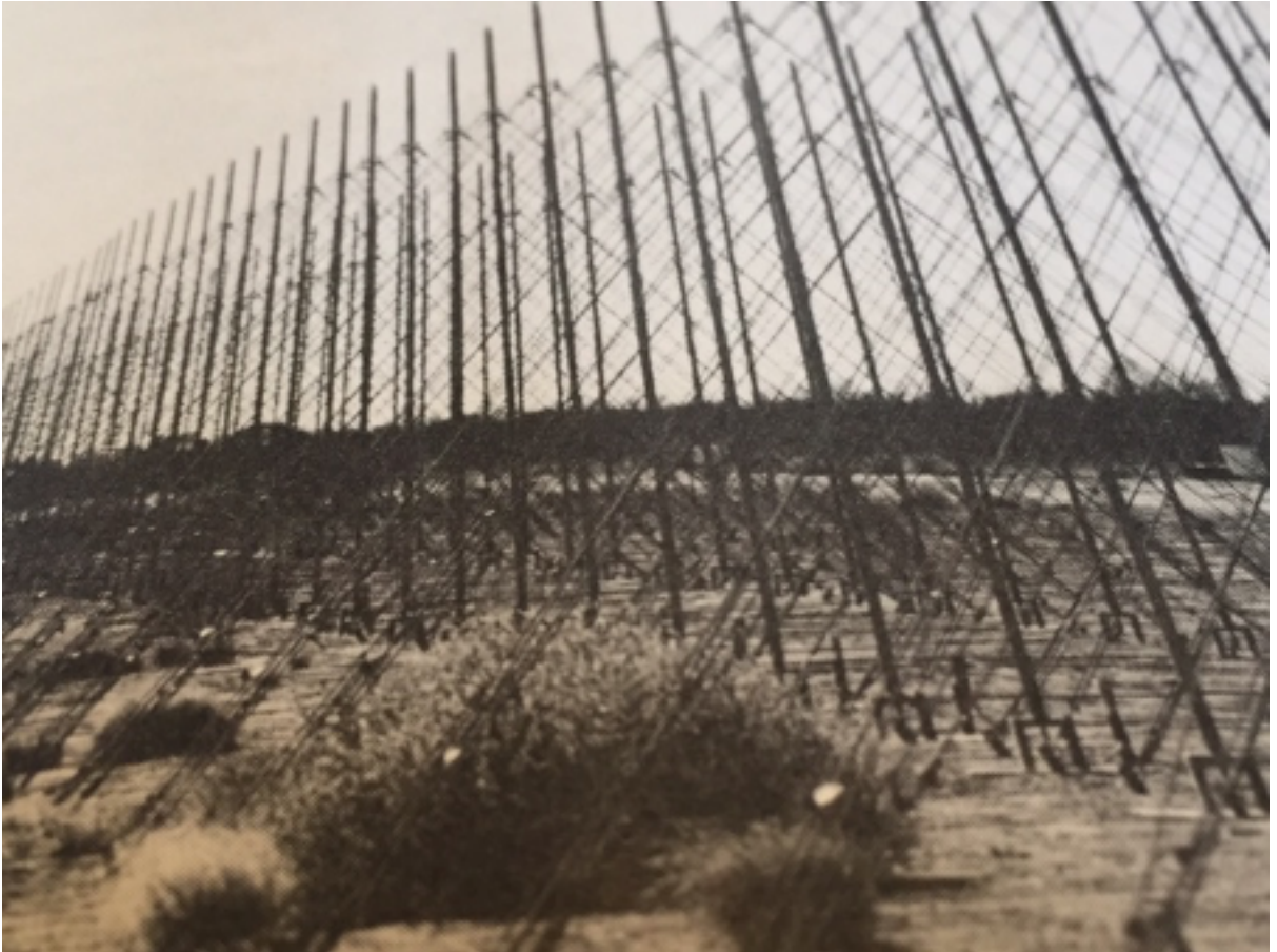
Figure 4: The aerial array of the Jindalee over the horizon radar. Source: 'The Defence of Australia', Department of Defence, 1987, p 35.
